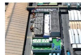
Installation Work and Progress of a Cooling Tower in Plant 1
