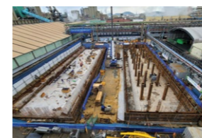
Plant 1 after the Completion of the Foundation Work
